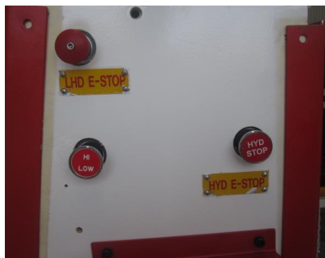
Hi-Low Valve fitted to console
