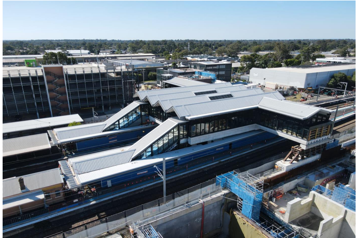
St Mary's Train Station Upgrade — progressed to c.95% completion at 30 June 2026
